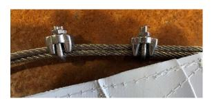
**Step 5** | Tighten tensioners until the cover is tight. Once tight set the lock nuts in place.
